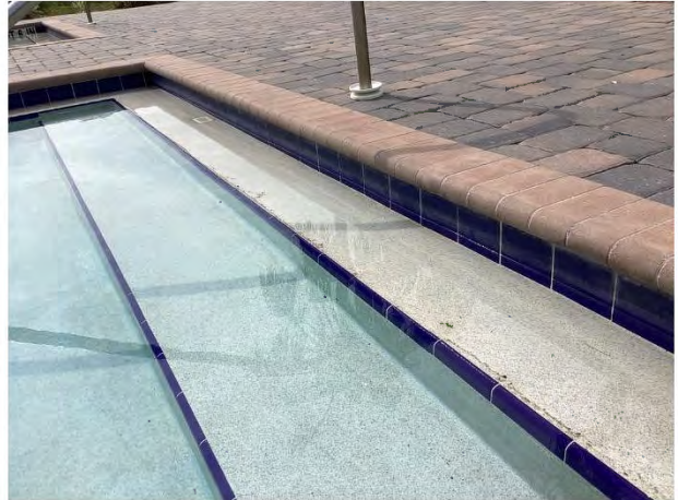
Pool plaster finish with tile perimeter
