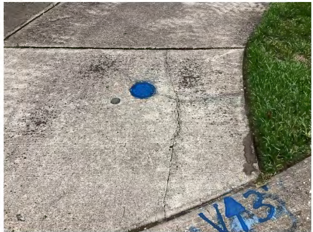
Sidewalk cracks
