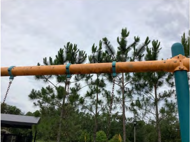
Equipment finish deterioration
