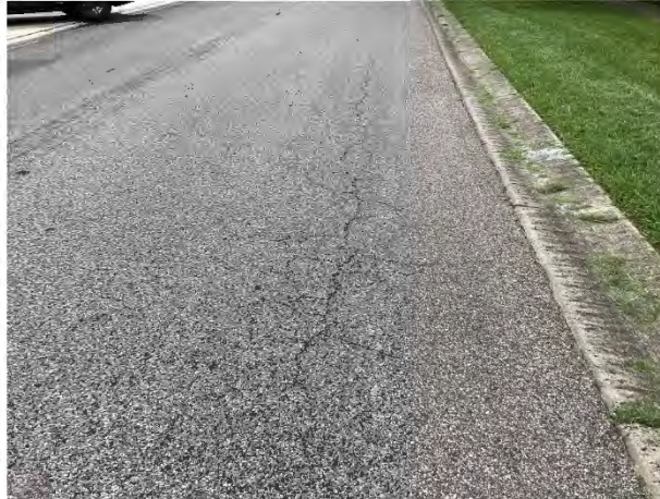
Pavement cracks
