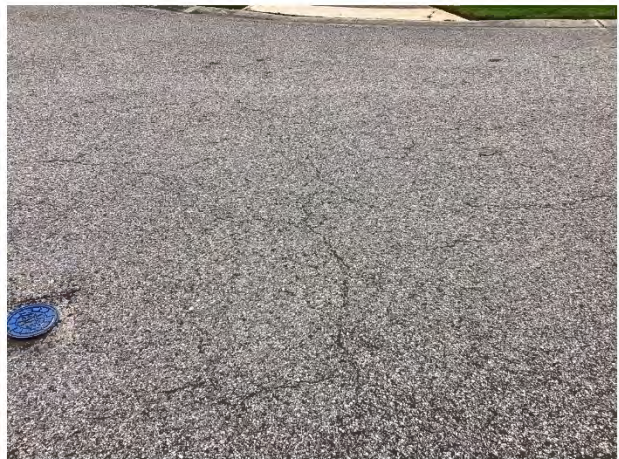
Pavement cracks
