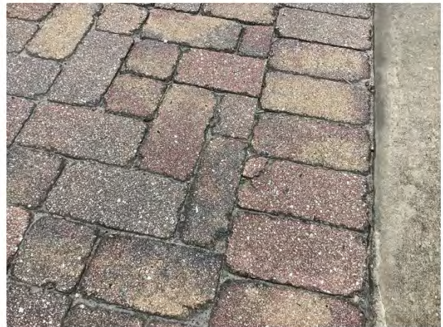
Paver cracks
