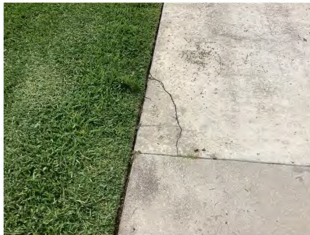
Sidewalk cracks
