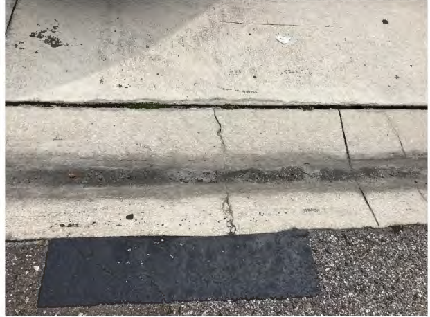
Concrete cracks
