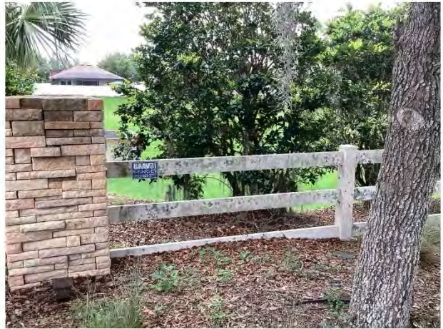
Fence finish deterioration
