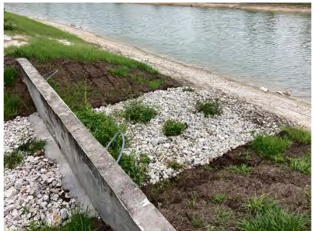
Shoreline remediation at pond control structure
