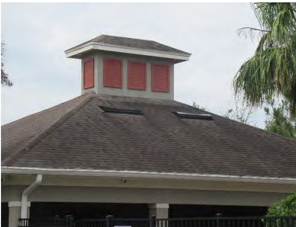
Clubhouse asphalt shingle roof (note weathering)
