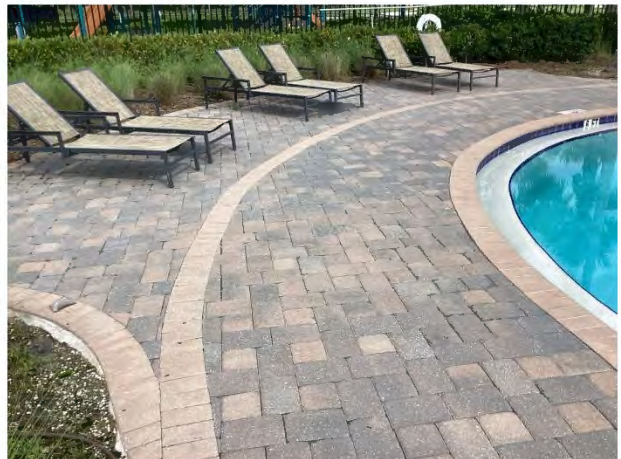
Paver pool deck overview
