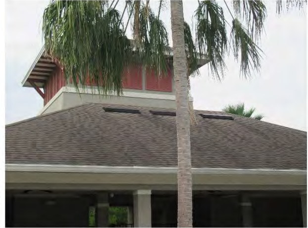
Clubhouse asphalt shingle roof
