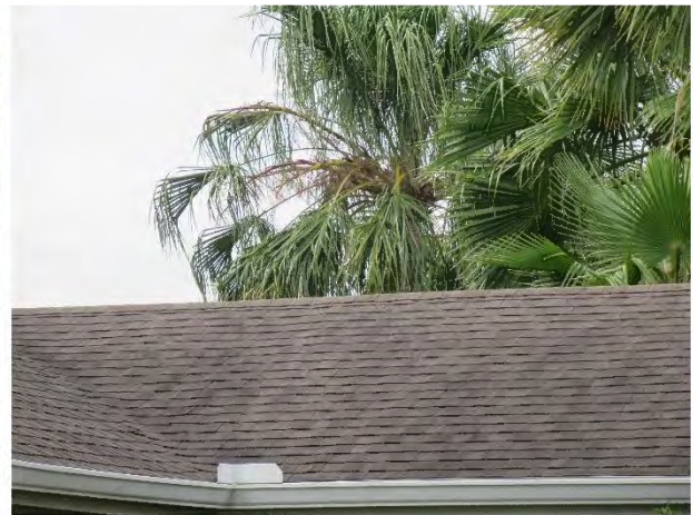
Clubhouse asphalt shingle roof
