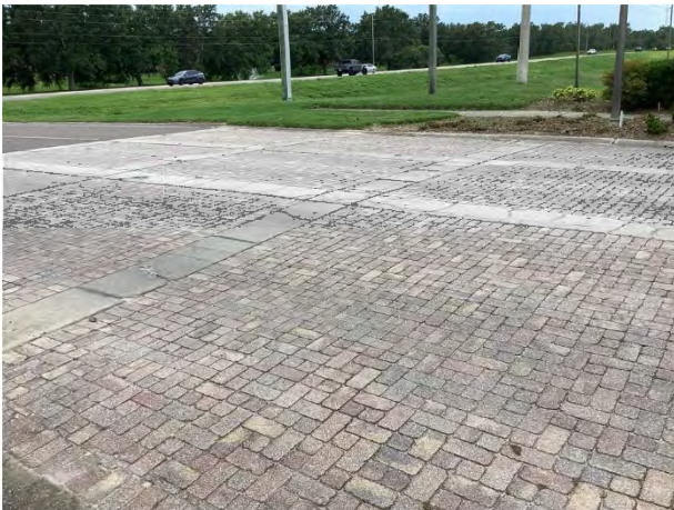
Masonry pavers overview
