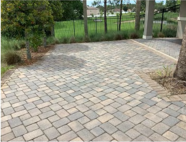
Paver pool deck overview
