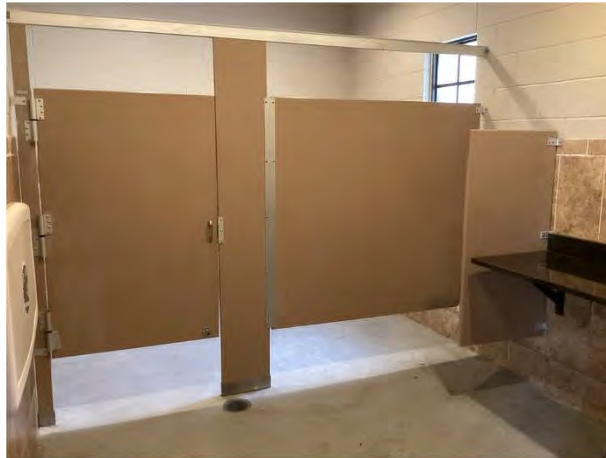
Rest room overview
