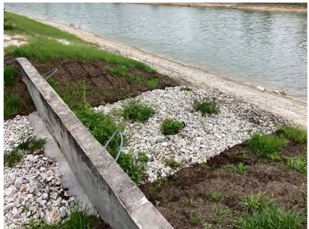
Shoreline remediation at pond control structure
