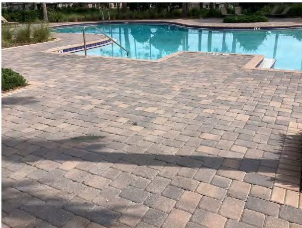
Paver pool deck overview
