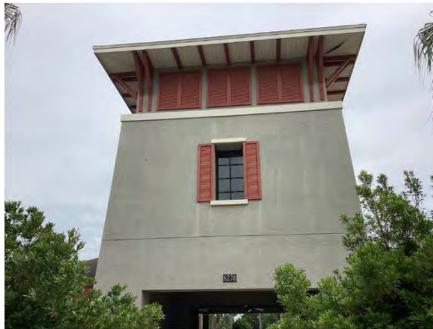
Stucco wall finishes
