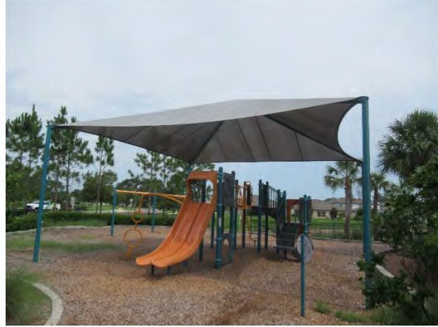
Shade structure overview
