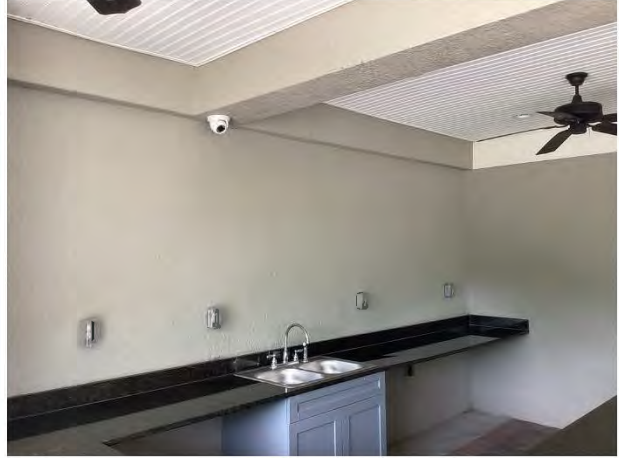
Stucco wall finishes
