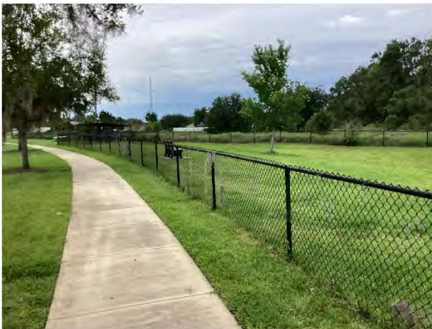
Chain link fence
