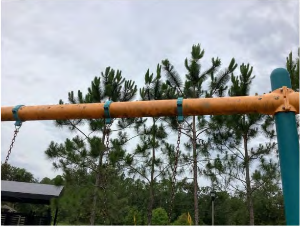
Equipment finish deterioration
