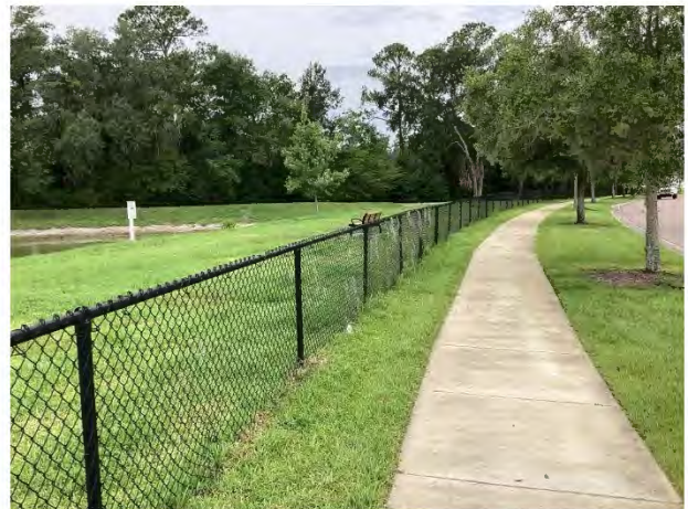
Chain link fence
