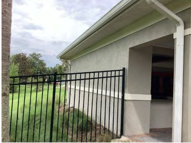
Stucco wall finishes
