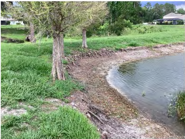
Minor shoreline erosion
